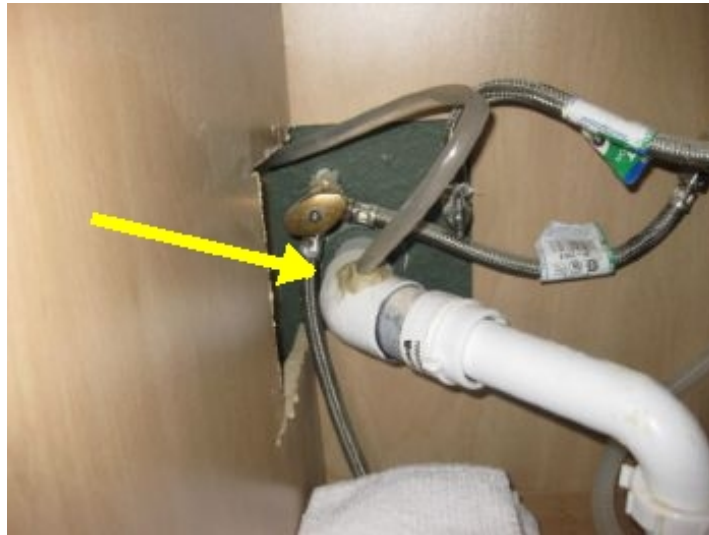
Ice maker improperly drained at bsmt. wet bar.
