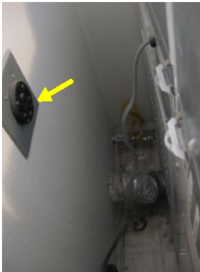
Dead dryer outlet and looped dryer flex vent.
