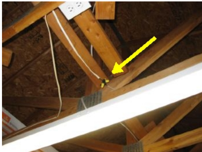
Exposed wire connection in garage attic.
