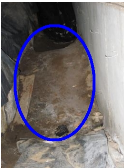
EWxpopped dirt and standing water in crawl space
