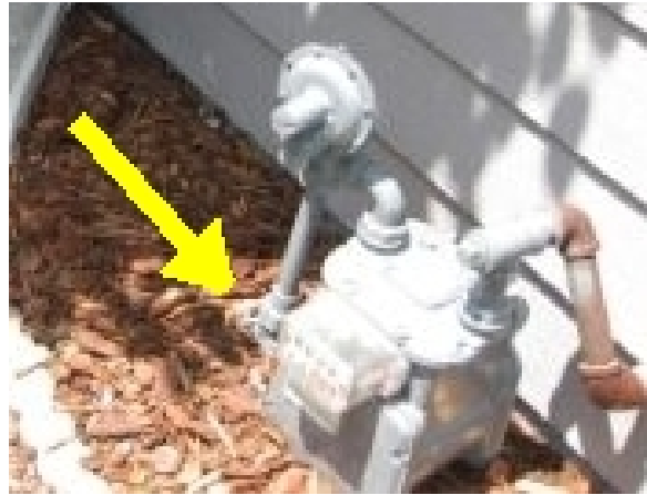
Main Gas Shut off
