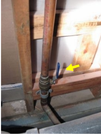
Main Water Shut off
