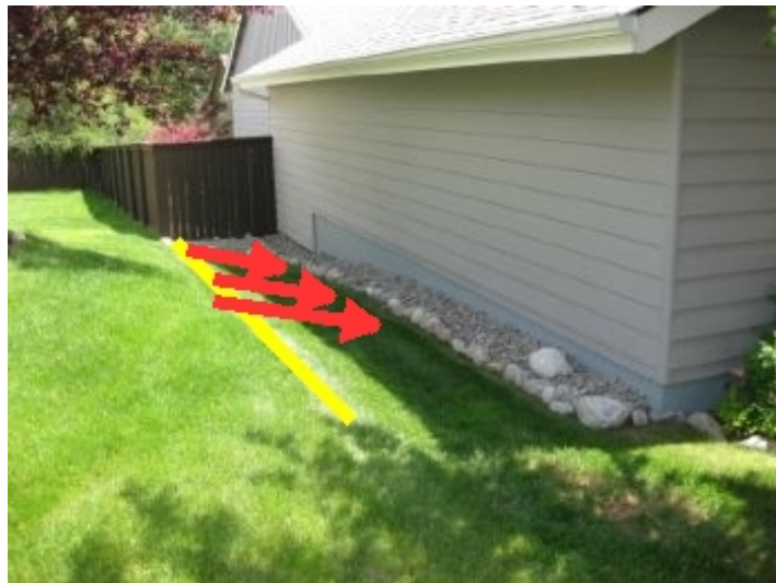
Negative slope contributes to damp crawl space.
