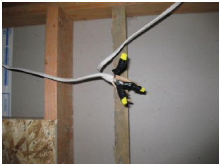
One of 3 similar exposed connections.
