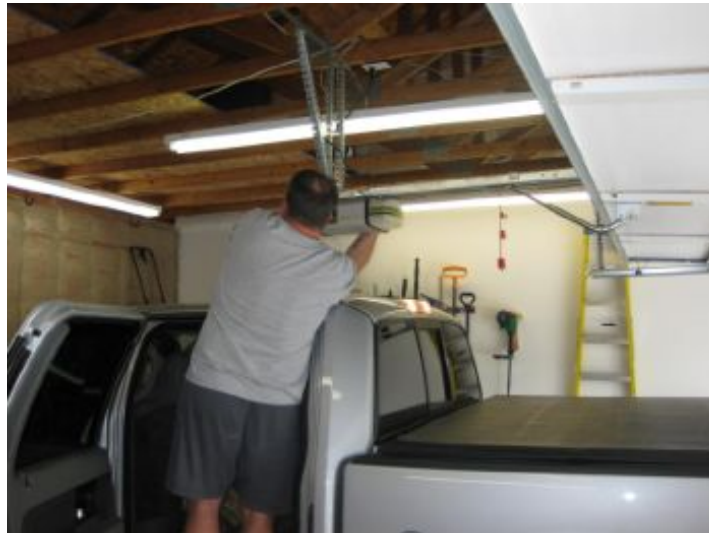
Garage door does not reverse with contact. Client attempting repair.
