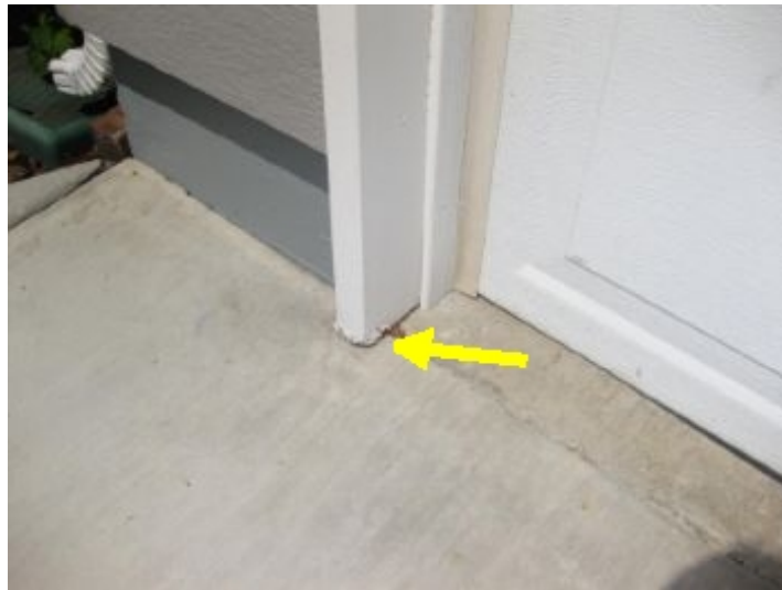
Trim wicking moisture and rotting.
